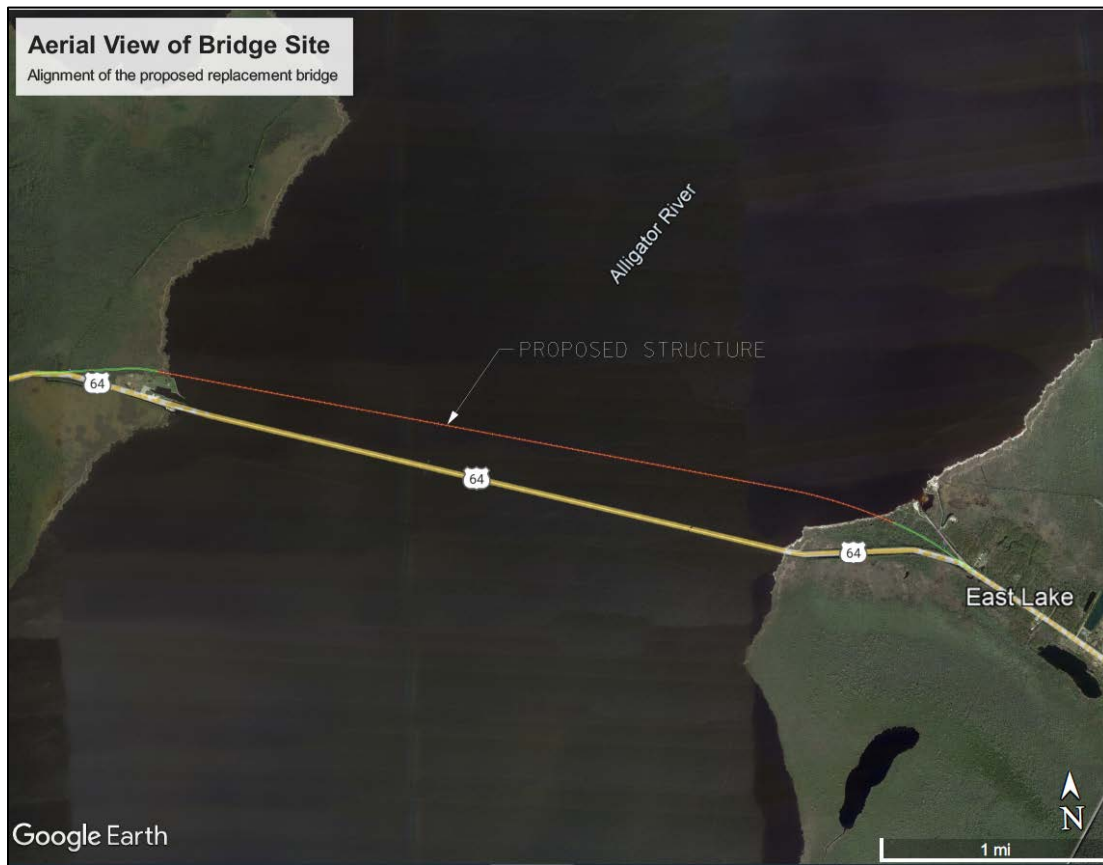
Figure 1-2: Aerial view of bridge site
